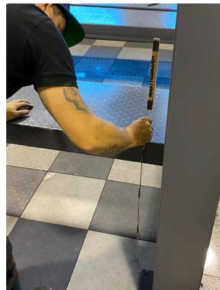
32. Raise the lifting ramps and place them on the bar at the same height in all corners. Adjust the latch steps if necessary and then tighten the wires.
