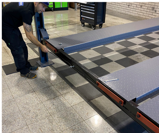
31. Fit the loop screw for the long linkage and thread it through.
