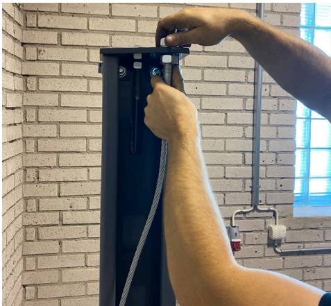
20. Secure the wires in the column but only so that the nuts have threads. They will be adjusted later therefore it must be space for adjustment.
